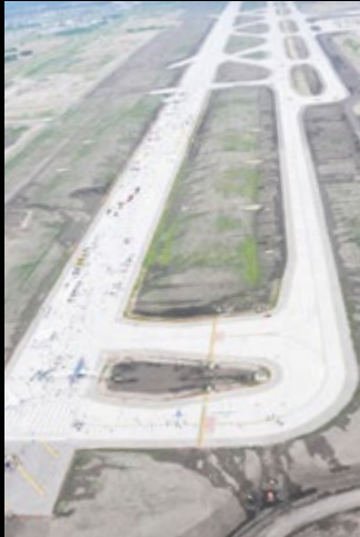
The runway, which is YYC's fourth runway, is 14,000 ft. long, 200 ft. wide and is the longest runway in Canada
