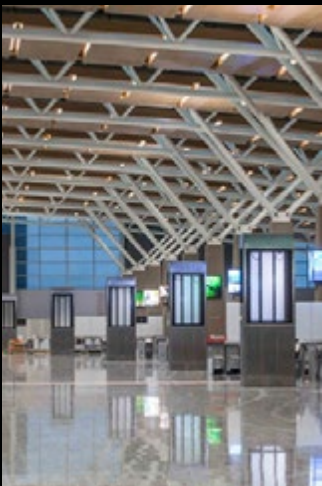
Canadian and U.S. Customs areas in Calgary's new International Terminal incorporate PABCO Gypsum's QuietRock sound deadening drywall, specified due to its high STC (Sound Transmission Class) ratings, even on closely spaced 20-gauge steel studs.
