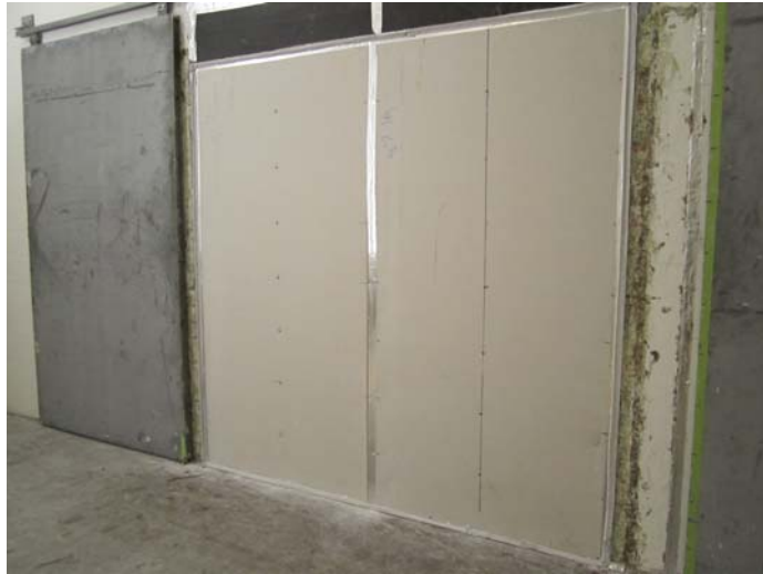
Figure 3: Receiving room side sheeting installed and sealed
