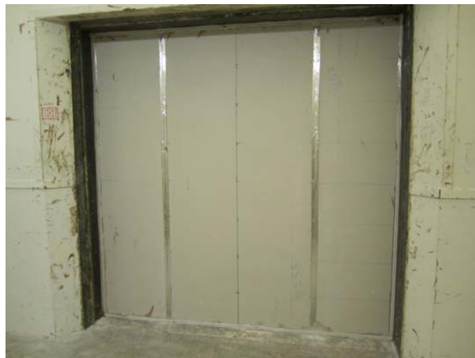
Figure 2: Source room side sheeting installed and sealed
