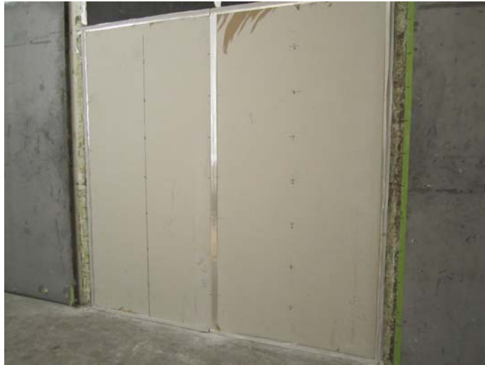
Figure 3: Receiving room side sheeting installed and sealed
