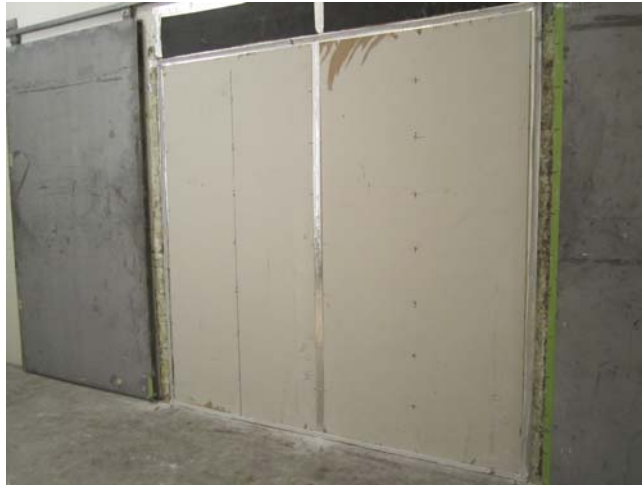
Figure 3: Receiving room side sheeting installed and sealed
