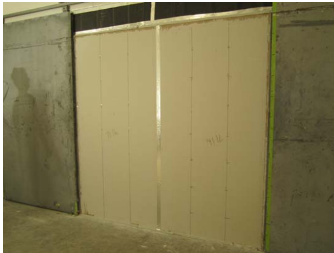
Figure 3: Receiving room side sheeting installed and sealed in the specimen opening
