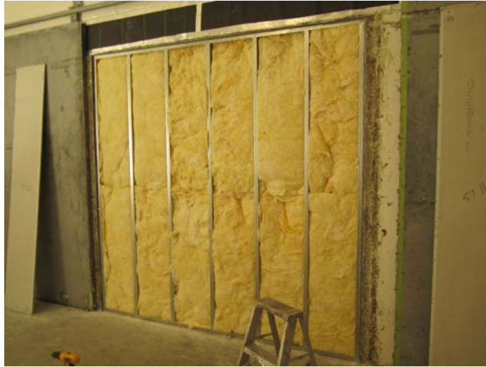
Figure 1: Insulated steel stud frame viewed from receiving room side
