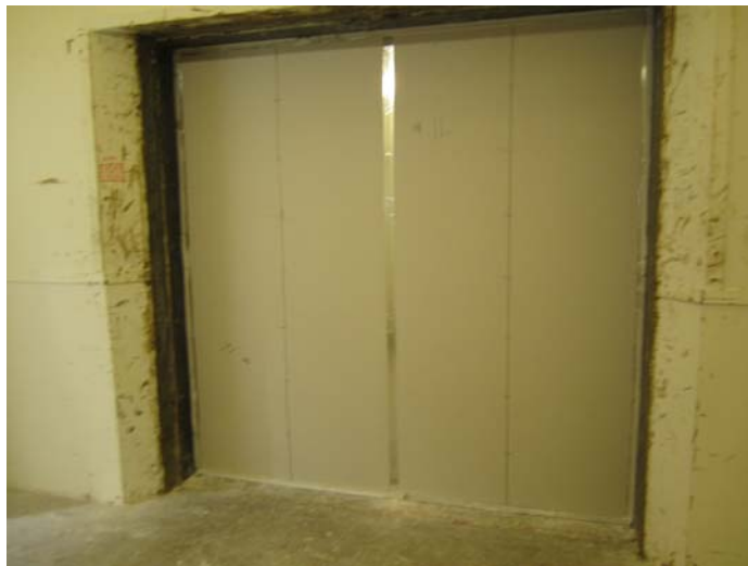
Figure 2: Source room side QuietRock ES installed and sealed in the specimen opening
